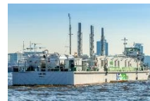
Cold Ironing Barge
