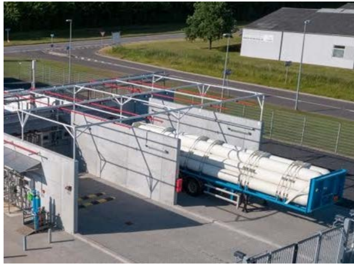
Figure 7: Representative trailer filling bay
