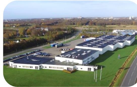
Denmark (Herning) H 2 Fueling Stations
